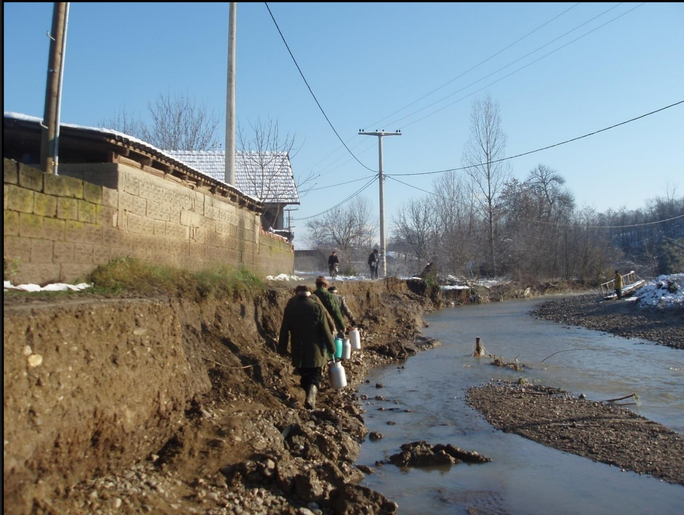
Destroyed local road
