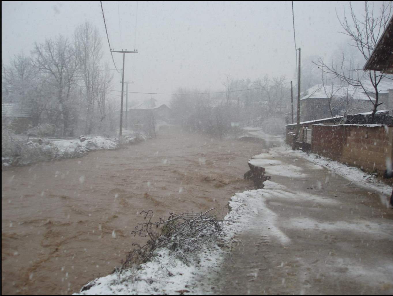
Destroyed local road
