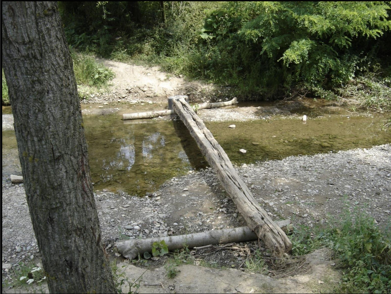
Improvised crossing over the river
