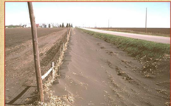
Destructive effects of wind erosion: Arable soil; Drainage / irrigation canal
