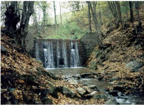
Figure 6. Check dam in the Bojkovački Potok torrent
