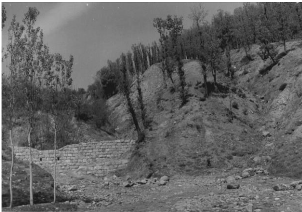
Figure 4. Check dam in the Panovljanska torrent
