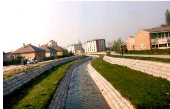
Figure 7. Regulation of lower course of the Štira torrent (Photograph: S.Kostadinov)
