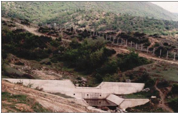
Figure 7 - Strait line check dam and arch line check dam - concrete
