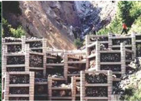
Figure 8 - Open check dam - Herheulidze type
