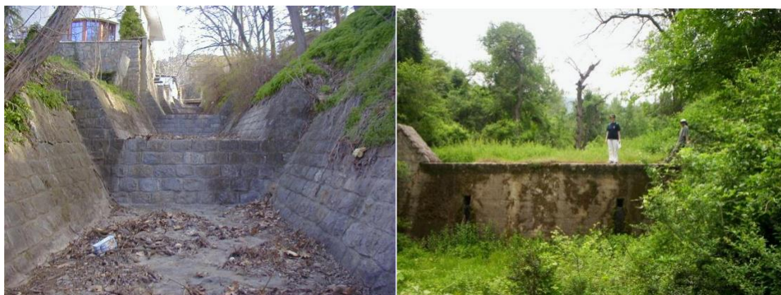
Figure 6- Channel and check dam in torrents on VodnoMounatin (50's – 60's of the XIX cent.)
