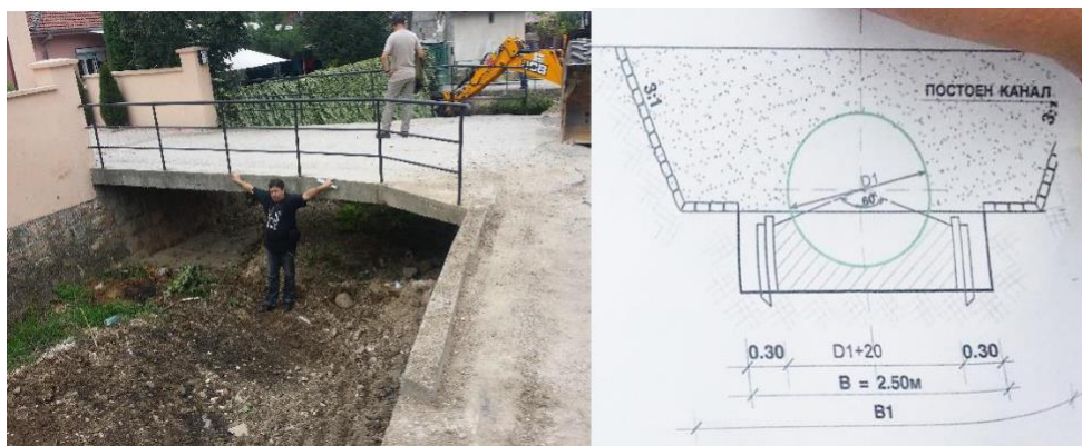
Figure 12 - Torrent bed designed by forest engineers in the 60's and extract form design for covering of the channel by civil engineer 2017 (wrong calculated maximal discharge even few years ago channel was full with water)
