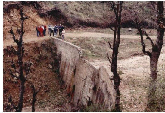
Figure 7 - Strait line check dam and arch line check dam - concrete
