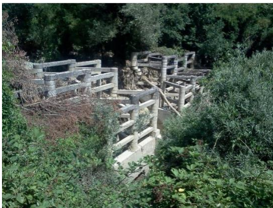
Figure 8 - Open check dam - Herheulidze type
