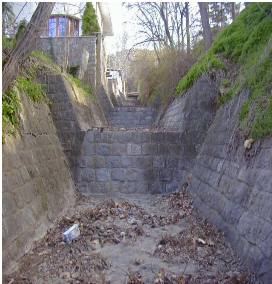
Channel and check dam in torrents on Vodno Mt. (50's – 60's of the XX cent.)
