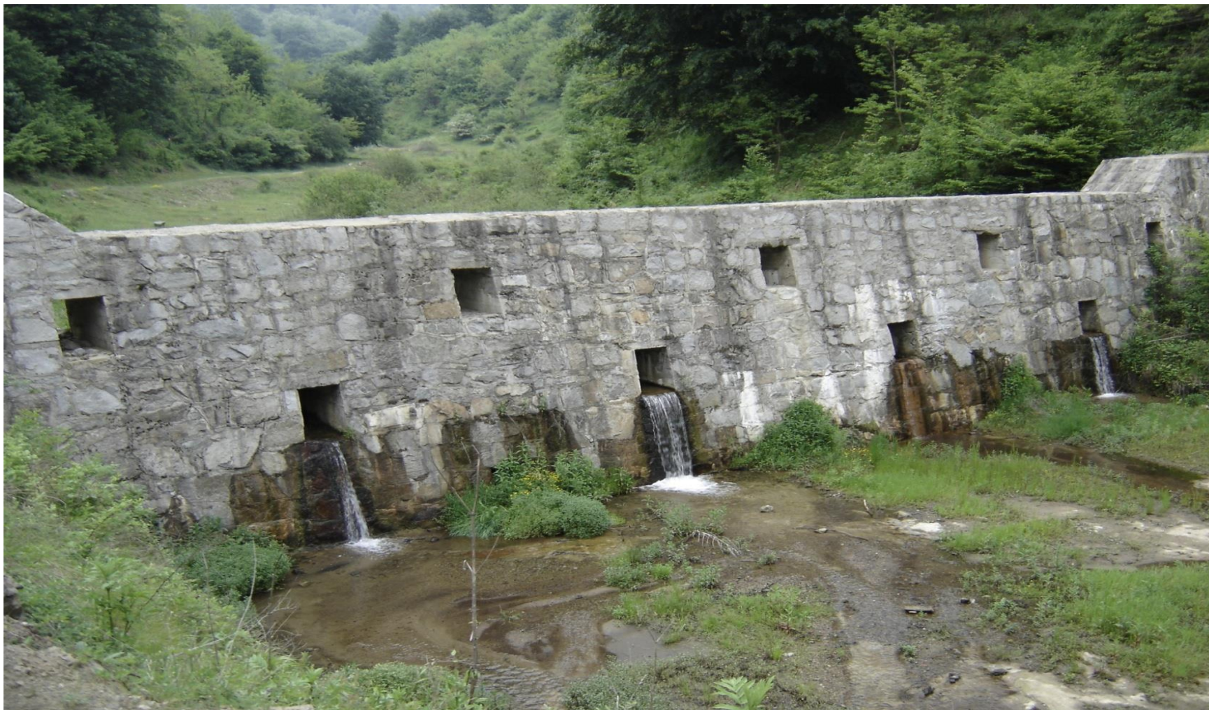
Stone masonry check-dam (2002)
