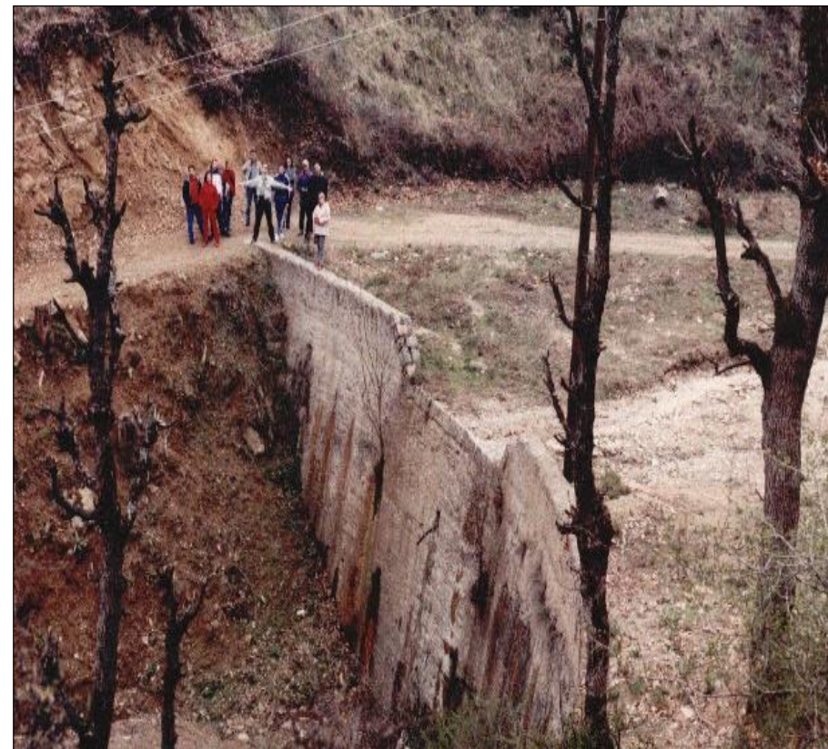
Straight line check dam and arch line check dam (concrete)
