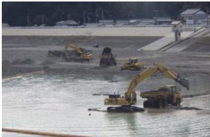
<Excavating the riverbed>
